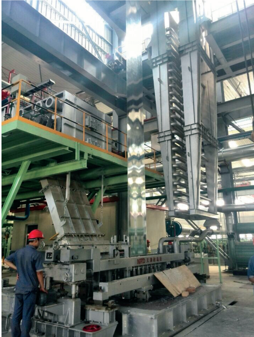
Galvanized Steel Factory
