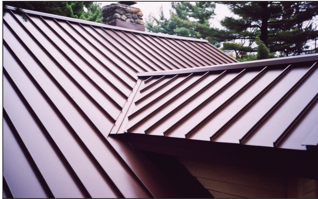
Galvanized Steel used for roofing
