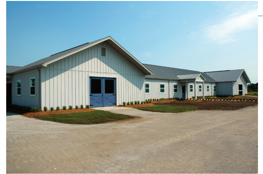
Galvanized Steel used for Agriculture (construction of barns)
